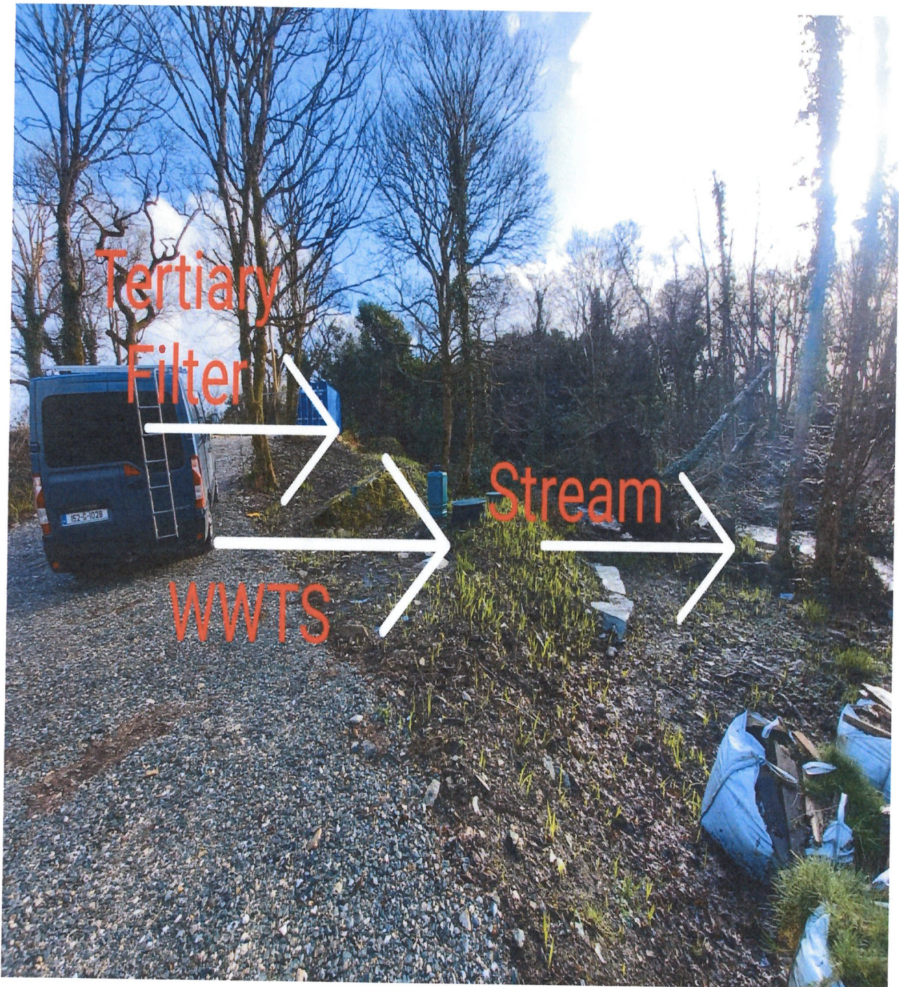
Figure 9.3 – View from the House Towards the WWTS and the Tertiary Filter Mound
